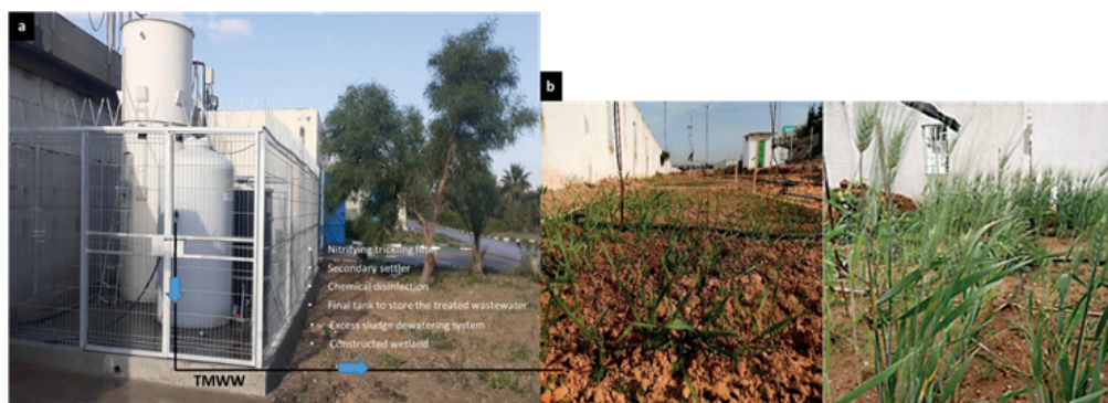
Figure 2- a) Municipal wastewater treatment process in Chotrana wastewater treatment plant (Ariana, Tunisia), b) Wheat irrigated with treated municipal wastewater using micro-sprinklers
