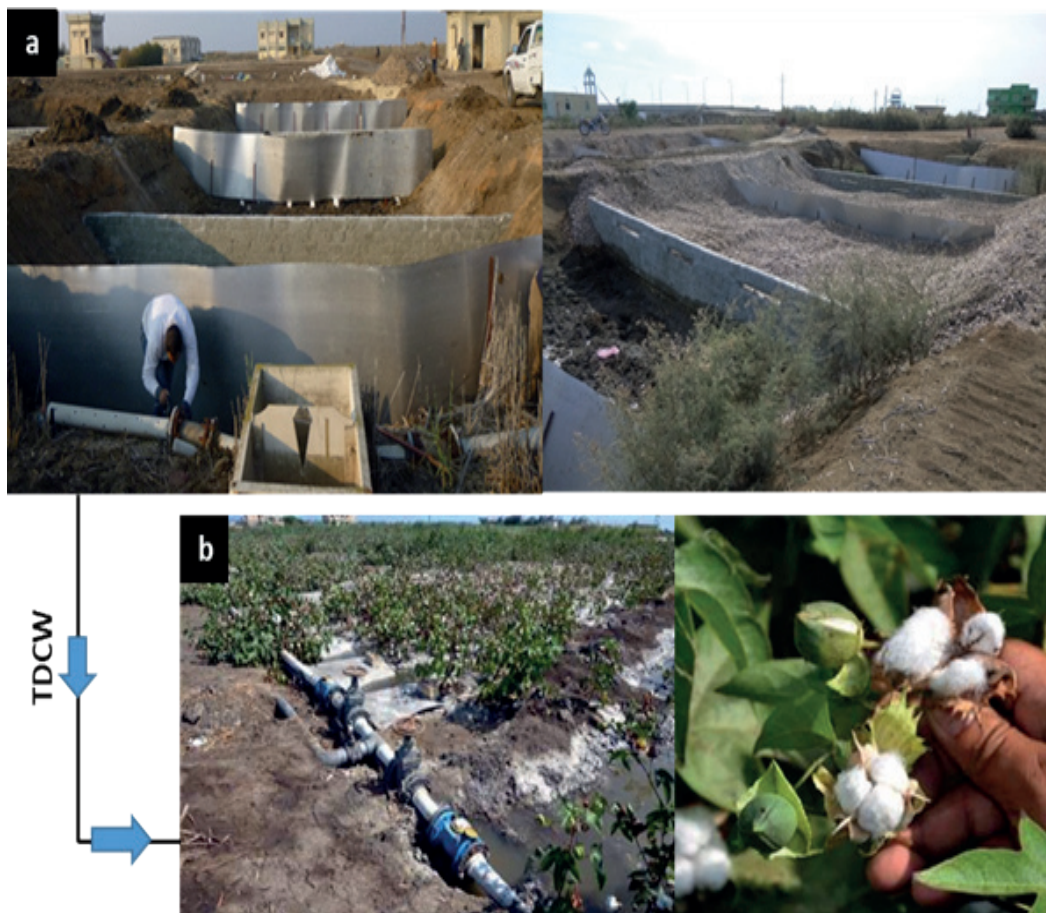
Figure 5- a) Drainage canal water treatment process in Lake Manzala in Egypt, b) Cotton plants irrigated with treated drainage canal water using gated pipes
